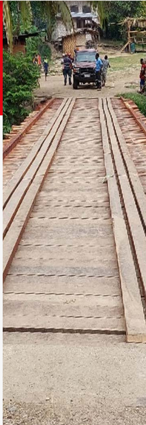
Neranda Bridge repairs, Hidden Valley
