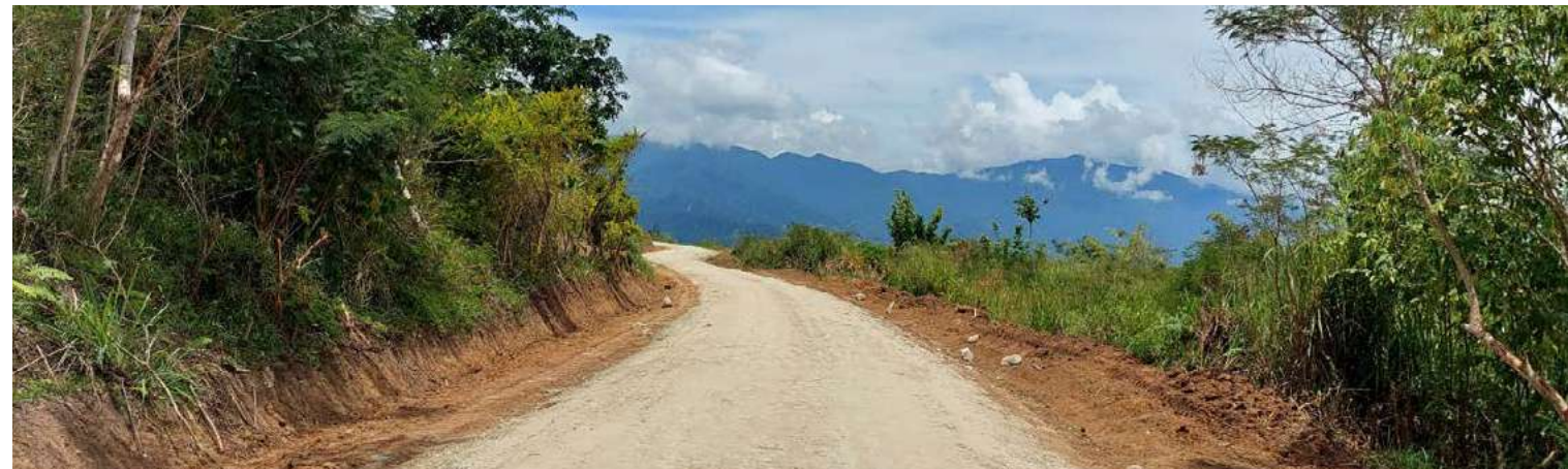
Nauti Road following maintenance, Hidden Valley Mine Community Roads
