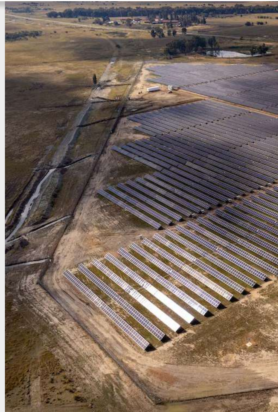
Tshepong renewable solar project
