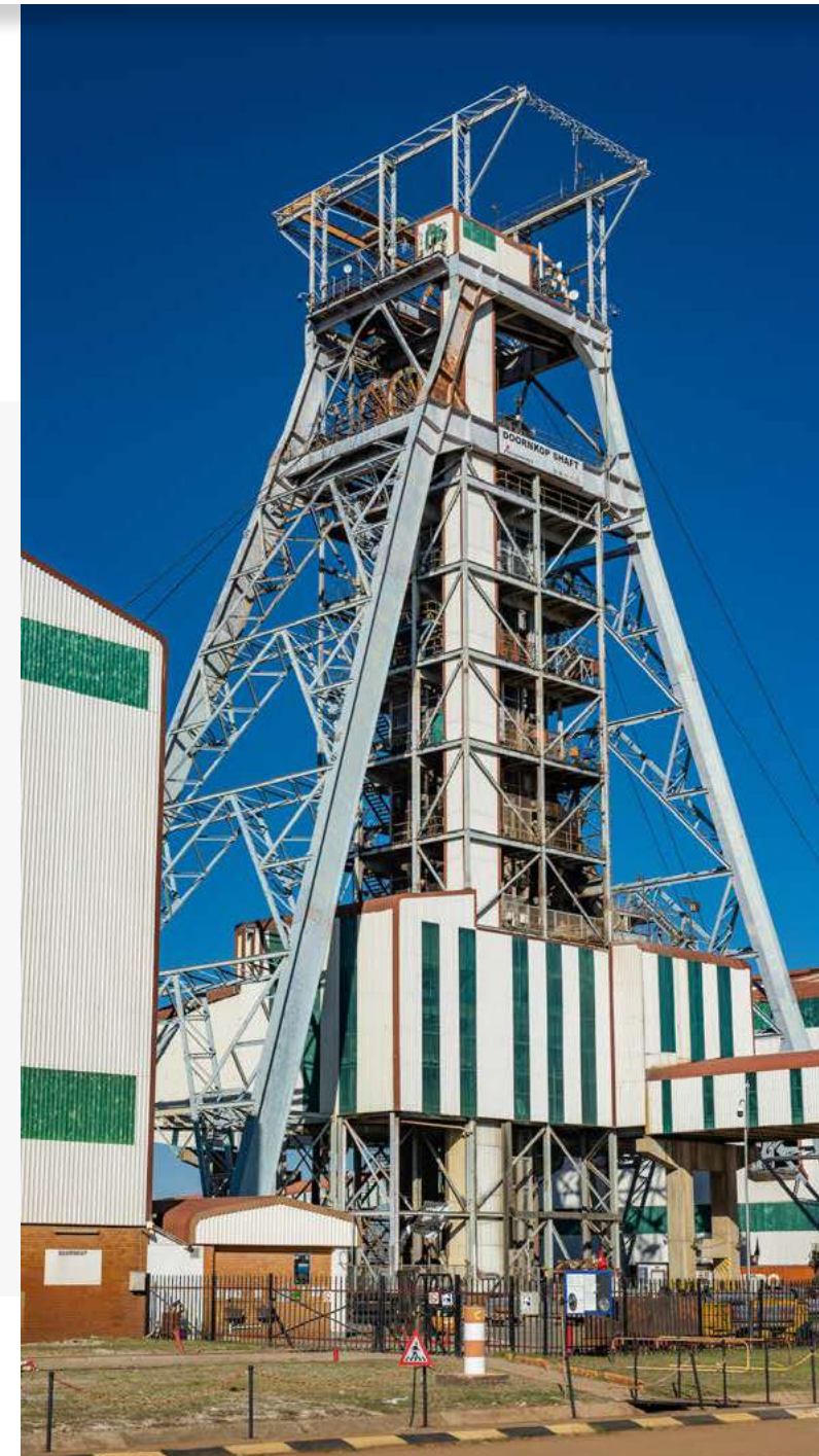
Doornkop shaft headgear
