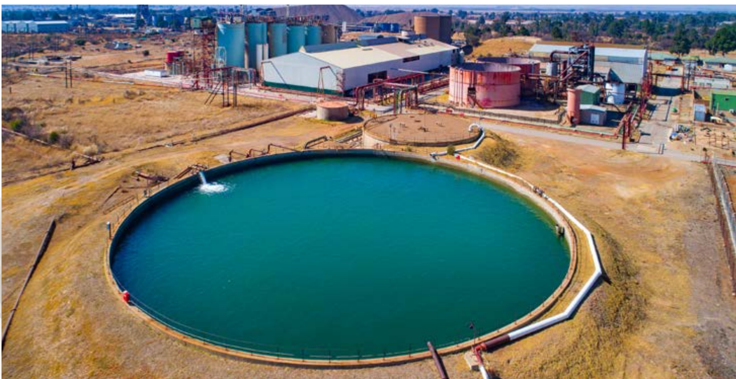
Mine Waste Solutions plant.
