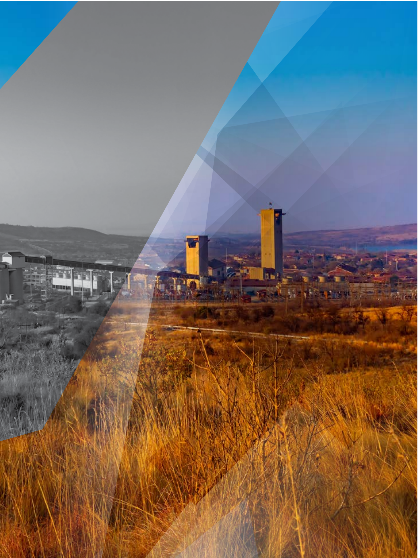
Main and service shaft head gear at Mponeng operations.
