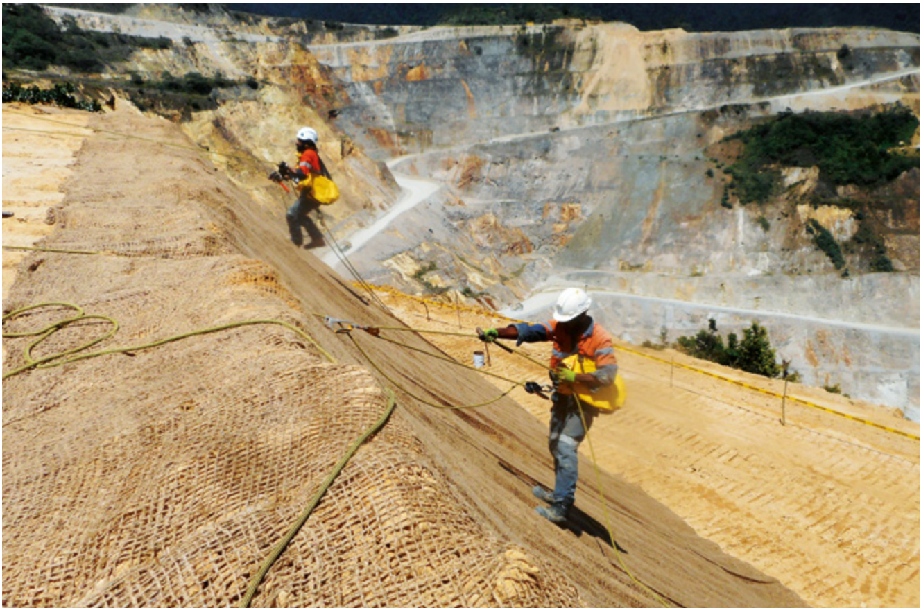
Steep slope rehabilitation
