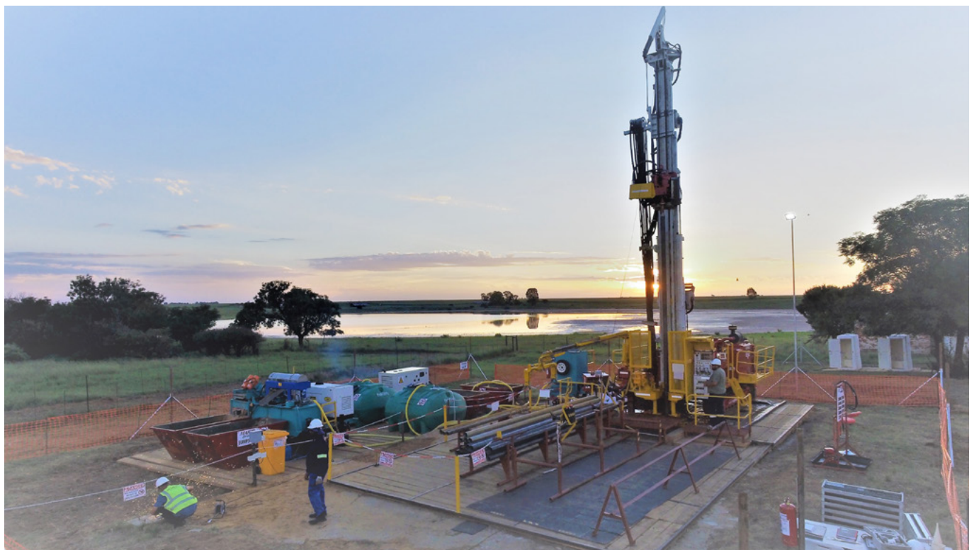
■ Target North – MAL 21 exploration borehole
