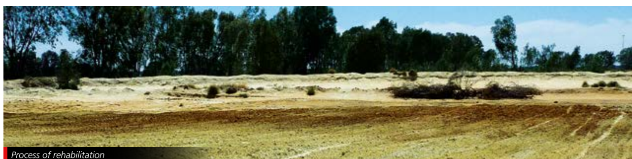
Process of rehabilitation
